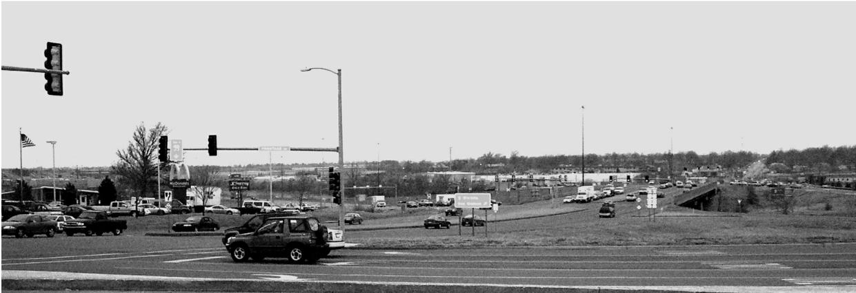
*A two-way frontage road (foreground) at an intersection with a cross street in Kansas City. Nearby I-35 runs beneath the cross street's overpass bridge (right). This intersection spacing is too close to the ramps to the interstate, and backups are common.*
